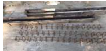
Figure 11. Beam moulds and reinforcement cages
