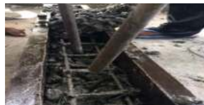
Figure 12. Pouring concrete into mould & compacting
