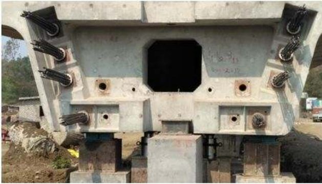
Figure 1: Cross Section Of Box Girder
