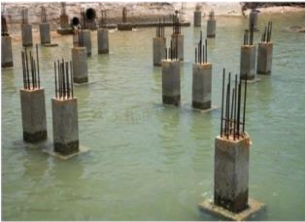
Figure 5: Modern Piling (Source: Rajesh, 2012)
