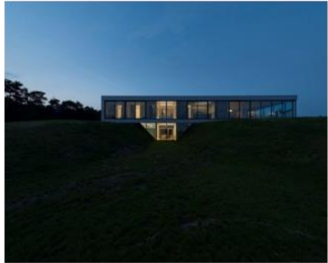
Figure 2: Terp Dwellings (Source: Architects, Jan 16, 2013)
