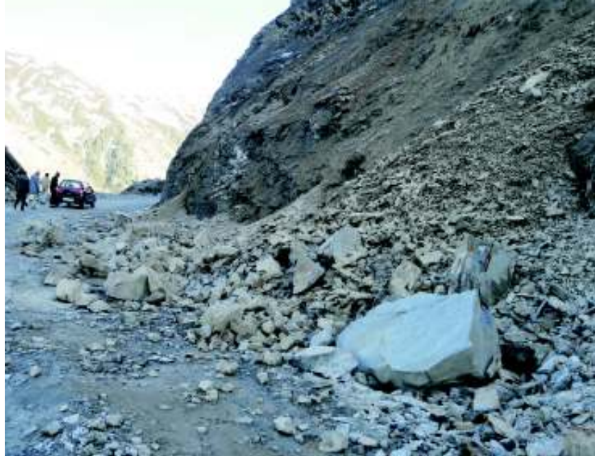
Figure 2: A Landslide Prone Area Along The Mughal Road Which Occurred Instantly As The Authors' Vehicle Crossed The Site
