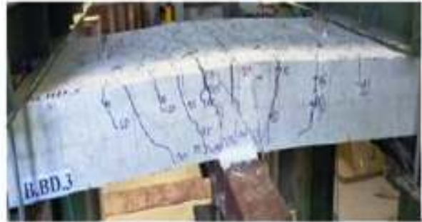
The bending failure of slab B.BD.3
