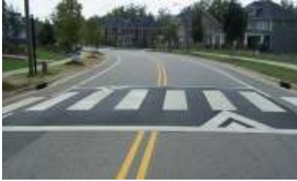
Fig. 8 Typical Example of Asphalt Speed Tables / Raised Crosswalk
