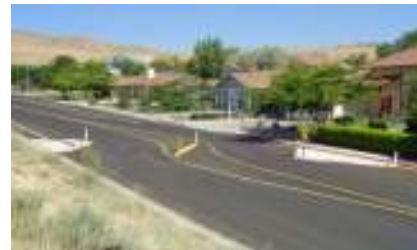
Fig. 3 Typical Example of Lateral Shifts
