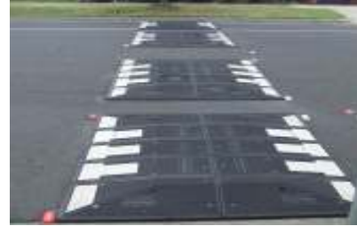
Fig 7 Typical Example of Speed Cushion
