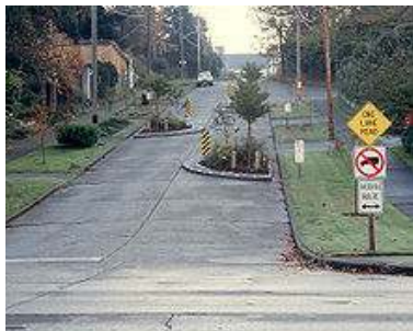
Fig. 2 Chicane used for the Traffic Calming
