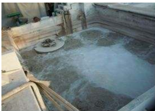
Figure 1b: Equalization tank
