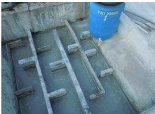
Figure 1a: Flocculation channel
