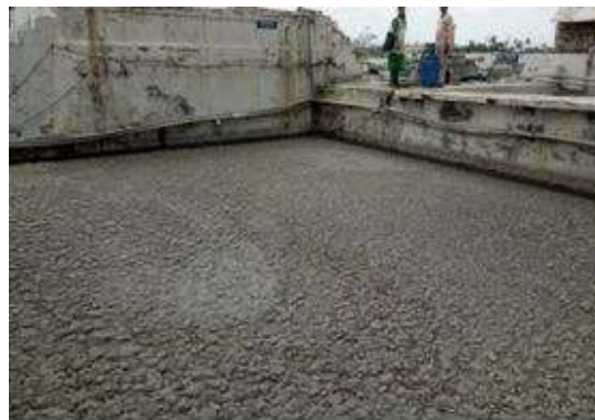
Figure 1d: Collection Tank
