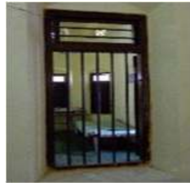
Figure 7: Window between master bedroom and guest bedroom
