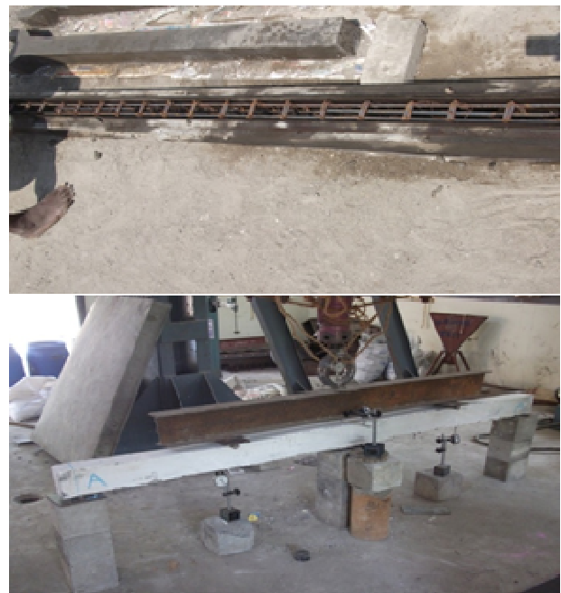
Figure 2.4: Casting of Beam
