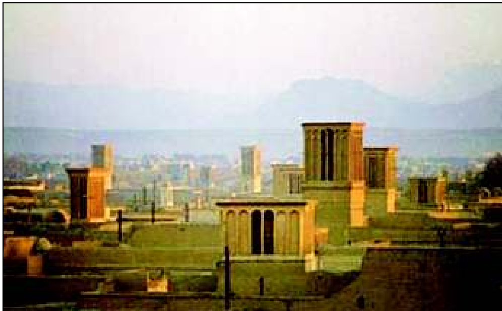
Figure 4 : Overview of the holes in Yazd
